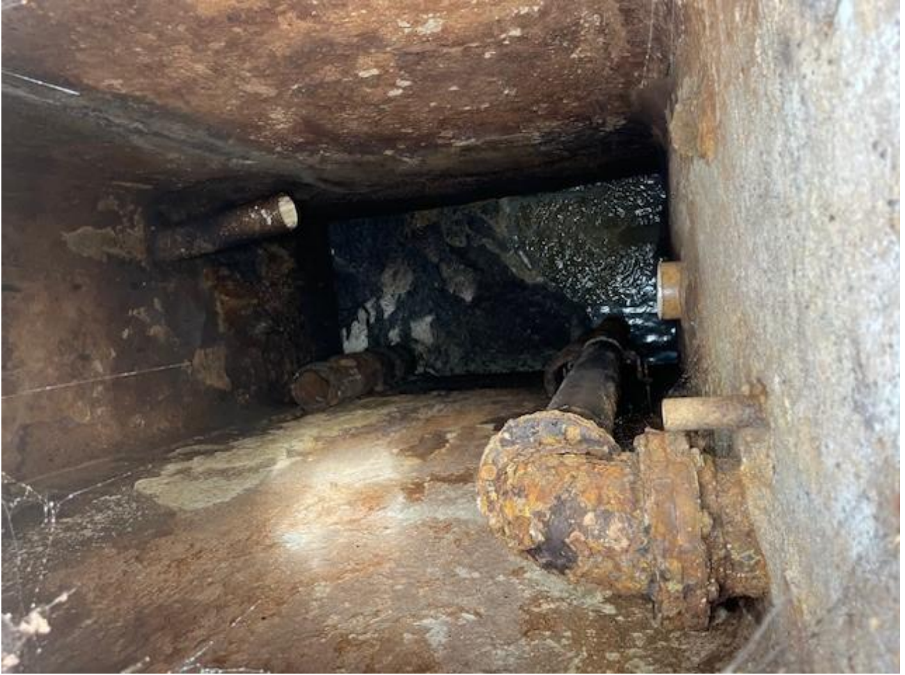
Lift Station No. 3 Wetwell – Pre Rehabilitation
