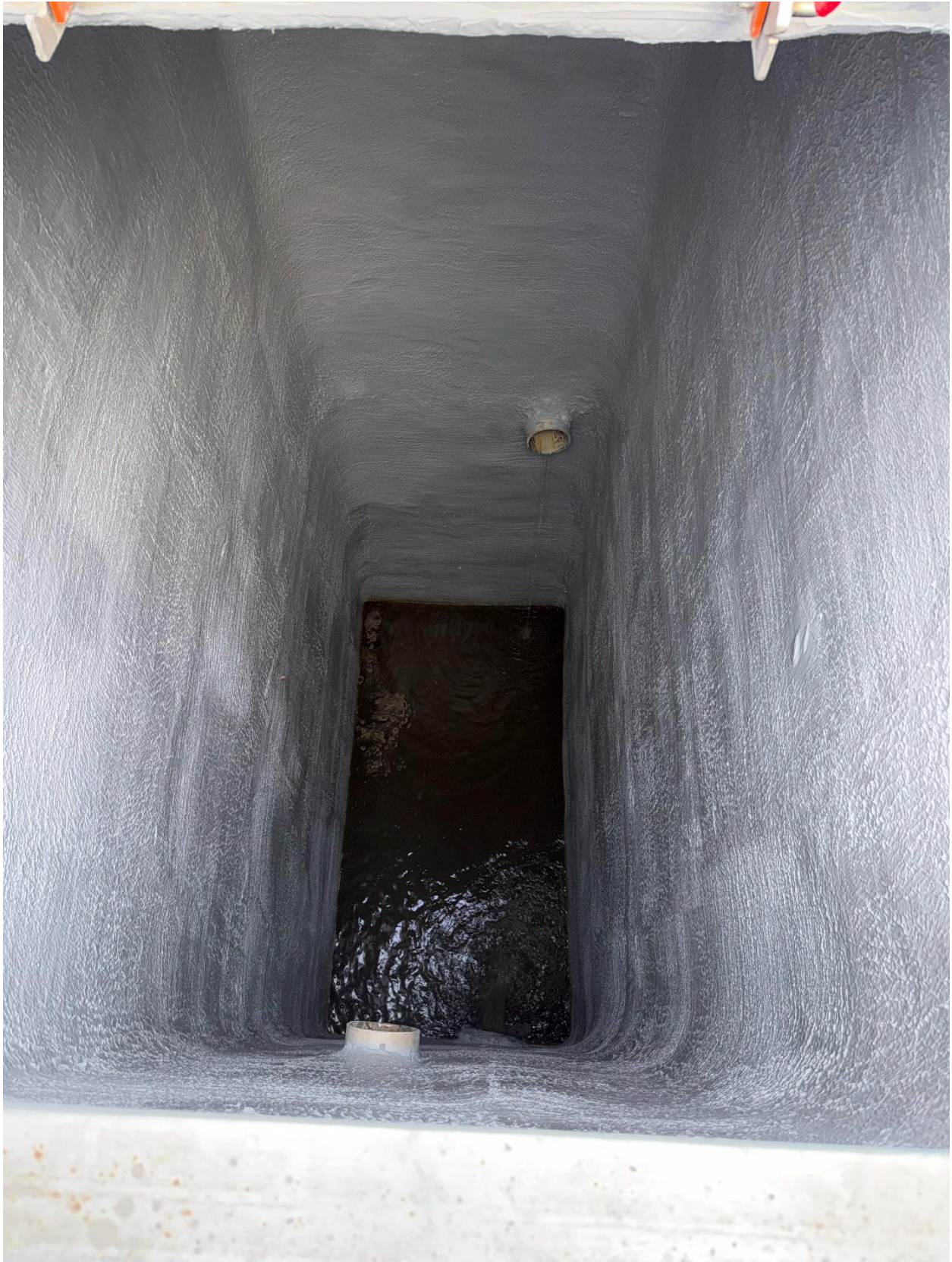
Lift Station No. 3 Wetwell – Post Rehabilitation
